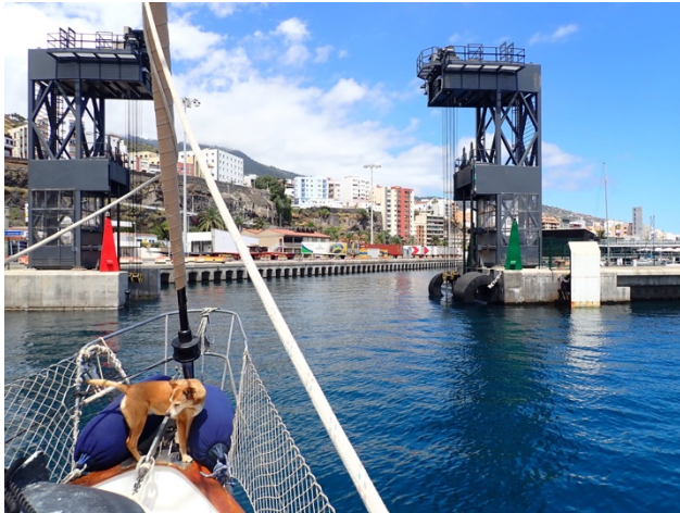
In Santa Cruz de La Palma, entry into the inner harbor requires close coordination with the local port authority, which must lower a steel door for a boat to pass. With the door lowered, the ocean swell inside the marina is quite persistent and uncomfortable. Once inside the marina and with the door raised, the water is flat and like glass.
