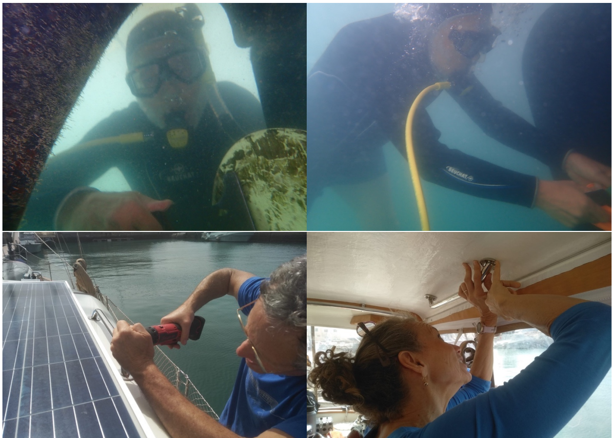
Never a shortage of work to do on a cruising sailboat. Here Juan and I are cleaning the bottom of plant and barnacle growth using our hookah rig, and Vicki and I through-bolt handhold rails inside and outside on the Bimini we installed in Menorca.
